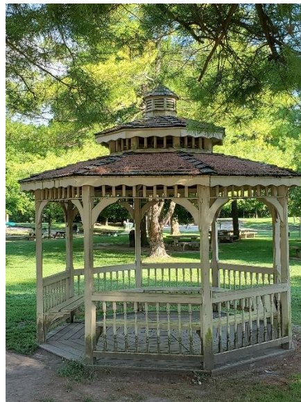
Existing Nisbet Park Gazebo
