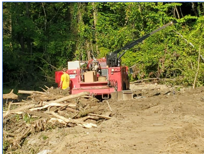
Insert-A-Valve Installation – Miamiview Drive Project
