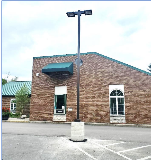
New Floodlight Installation – City Hall Parking Area
