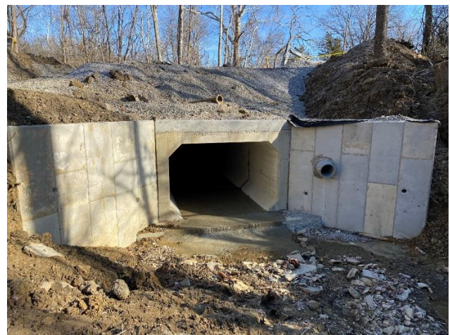
Miamiview Drive Culvert - After
