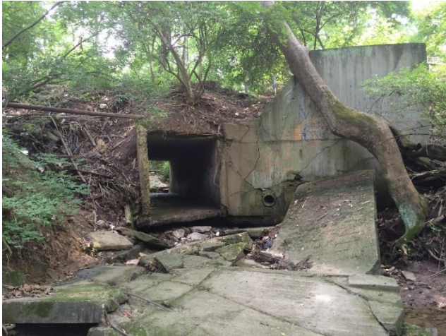
Miamiview Drive Culvert – Before
