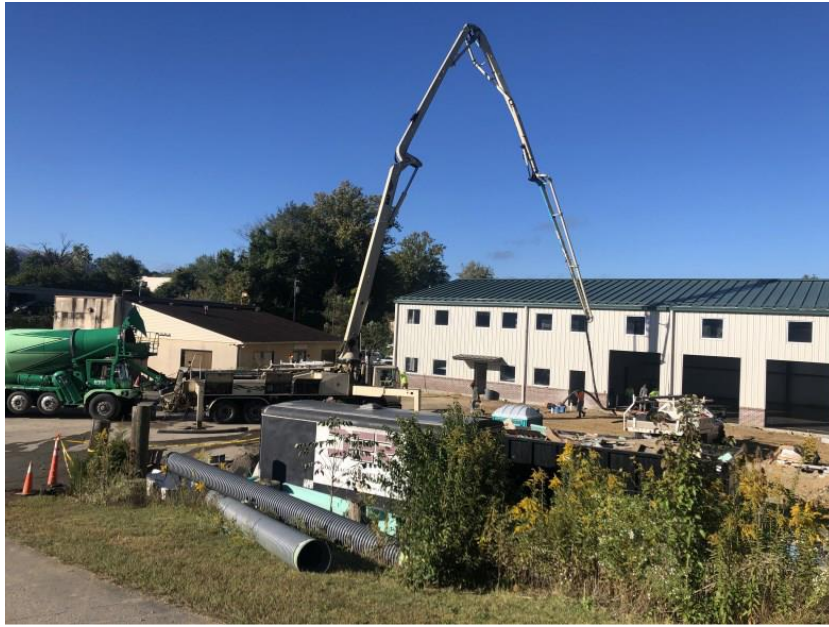
Concrete Slab Installation at New Public Works Building
