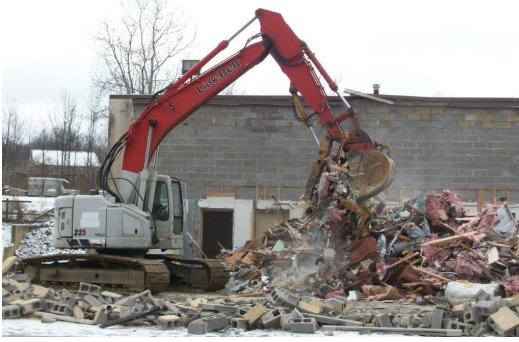
The old Public Works office building was demolished this week.
