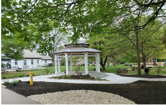
Nisbet Park Gazebo gets finishing touches
