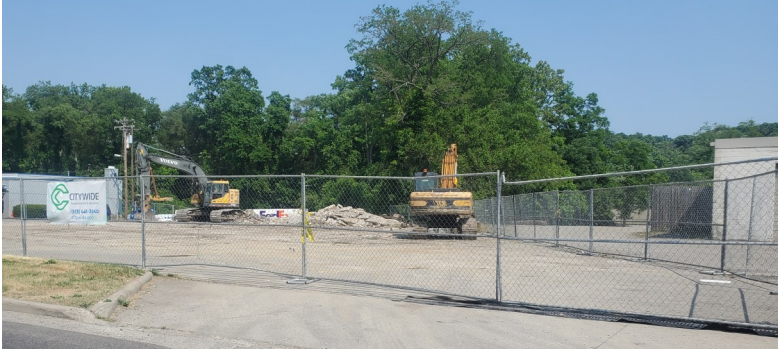
Vacant structure at 501 Loveland Madeira Road is razed
