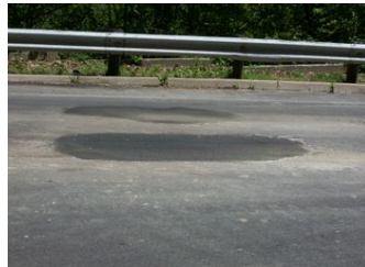
W Loveland Water Leak Repair 1
