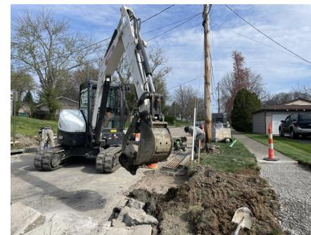
Progress continues on the Cherokee Water Main Project, with several key tasks completed this week. Waterline work included testing and purging along the stretch from Sunrise Drive to West Main Street, and on West Main from Cherokee Drive to Highland Street. Service lines and meters were installed between Sunrise and West Main, while crews continued installing the 8-inch waterline from Tuscarora Drive to West Loveland Avenue.
